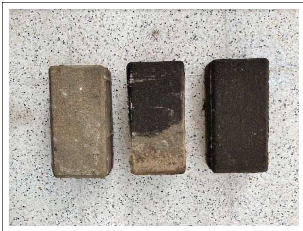
Figure 3. Concrete paving stones in different conditions.
