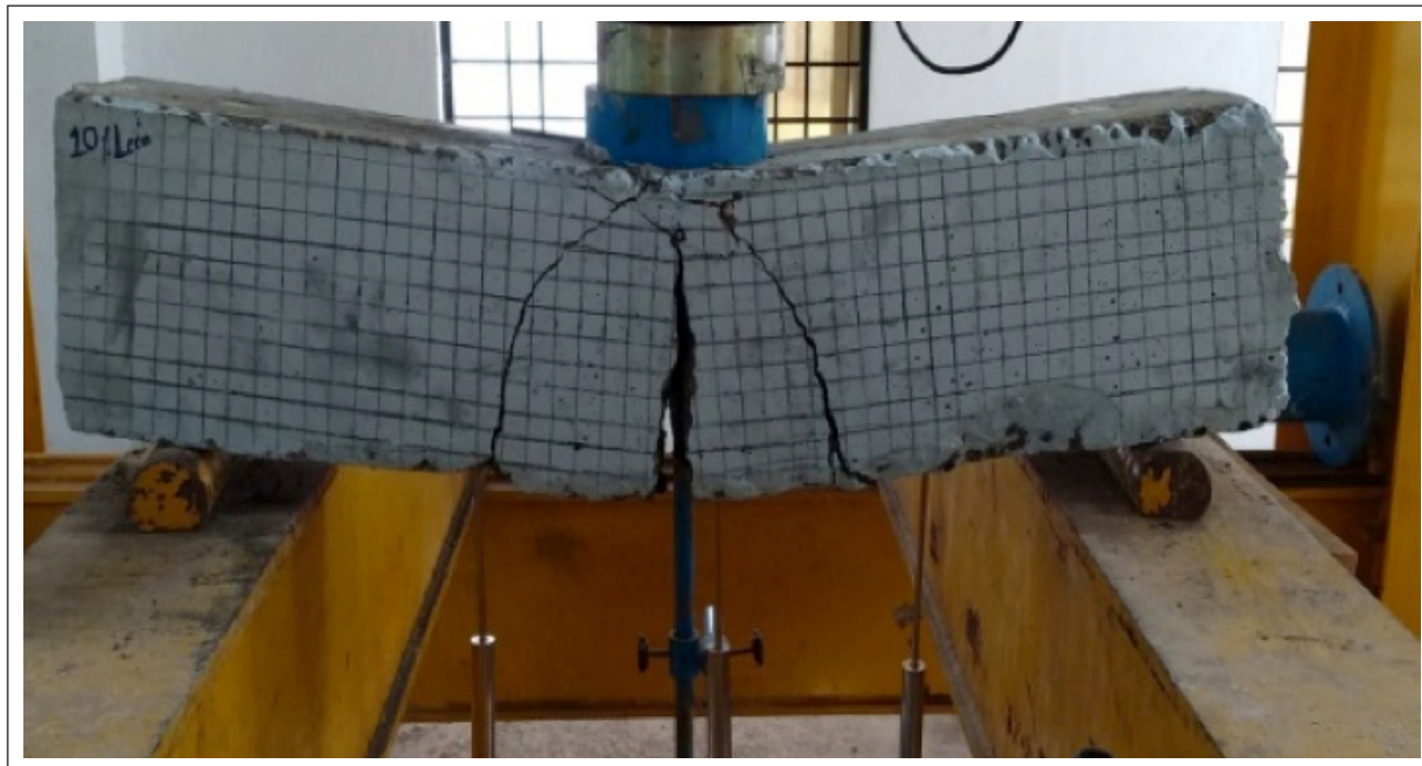
Figure 8. Crack pattern of beam LECA 5.
