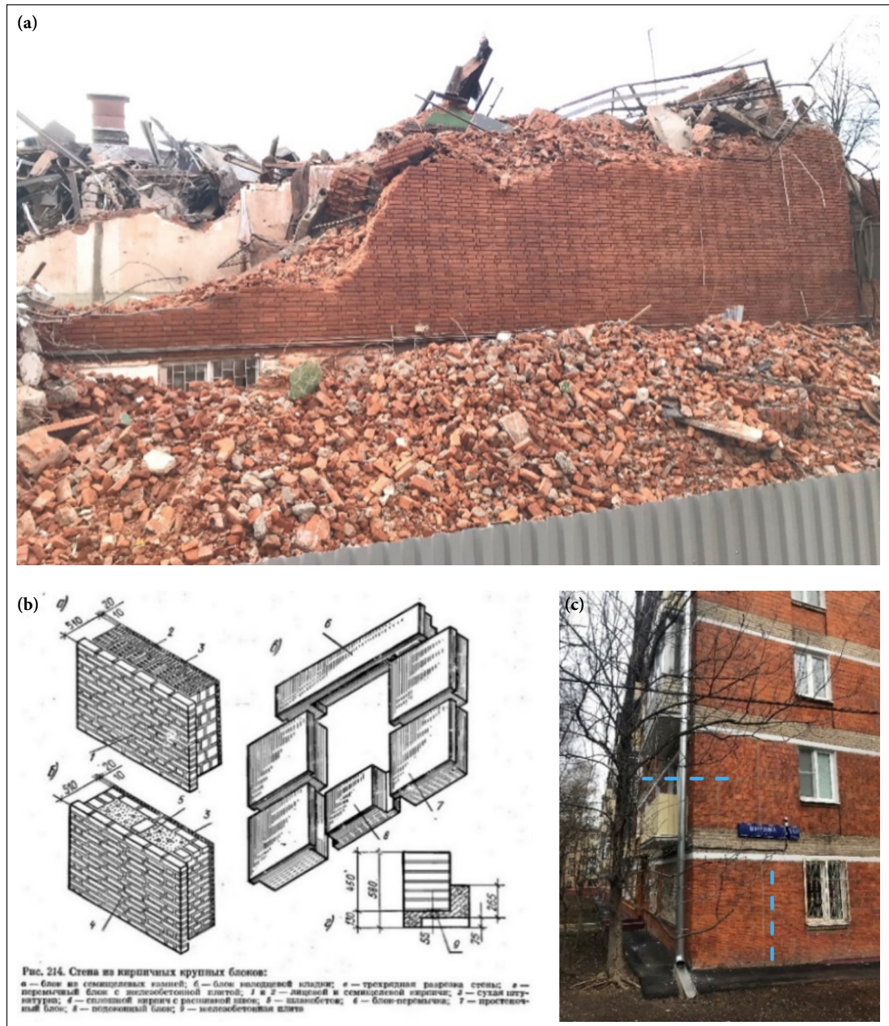
Figure 5. (a) The Vityaz Movie Theatre's brick walls were captured during demolition. (b) Schematic drawing illustrating construction with pre-built large masonry-block wall panels [38]. (c) The five-story mass housing project was constructed with prefabricated large-block brick wall panels in the 1960s–70s Moscow.
