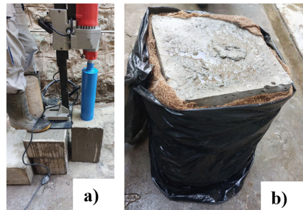
Fig. 2. a) Core sampling operation from a concrete column, b) wet curing of specimens.
