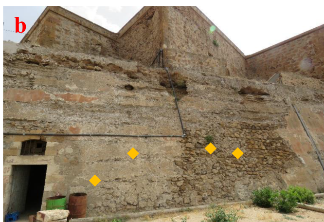
Fig. 1. Example of some of sampling areas (mentioned in Orange) selected to obtain and drill mortar samples: two photos above from elevation south west and North west, interior facade (a); exterior facade (facing the sea) (b).
