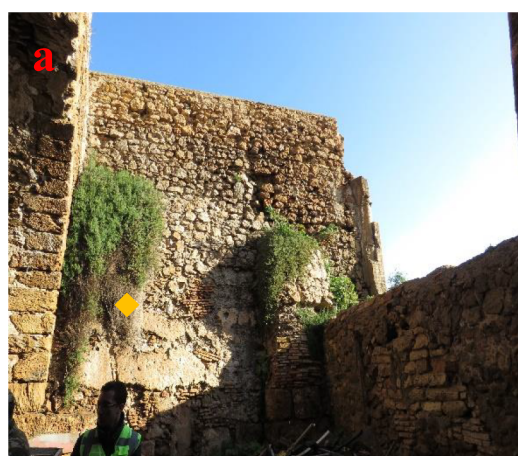
Fig. 1. Example of some of sampling areas (mentioned in Orange) selected to obtain and drill mortar samples: two photos above from elevation south west and North west, interior facade (a); exterior facade (facing the sea) (b).
