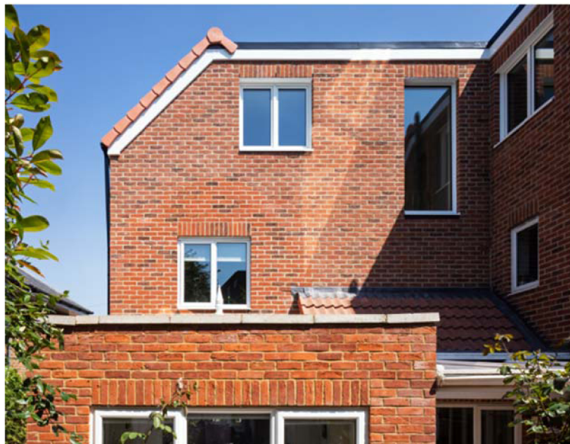
Fig. 8. External façade of Bathgate Road featuring clay brickwork and high-spec insulated cavity construction.
