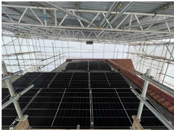
Fig. 4. Photovoltaic (PV) panels were installed during the Wimbledon loft conversion, demonstrating the integration of renewable energy technologies in line with the UK Future Homes Standard and sustainable design targets. 41 Seymour Road project.
