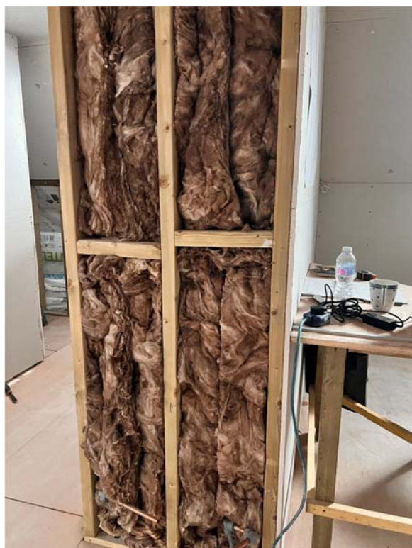
Fig. 10. Timber frame construction showing mineral wool insulation during on-site installation at Wimbledon loft conversion.
