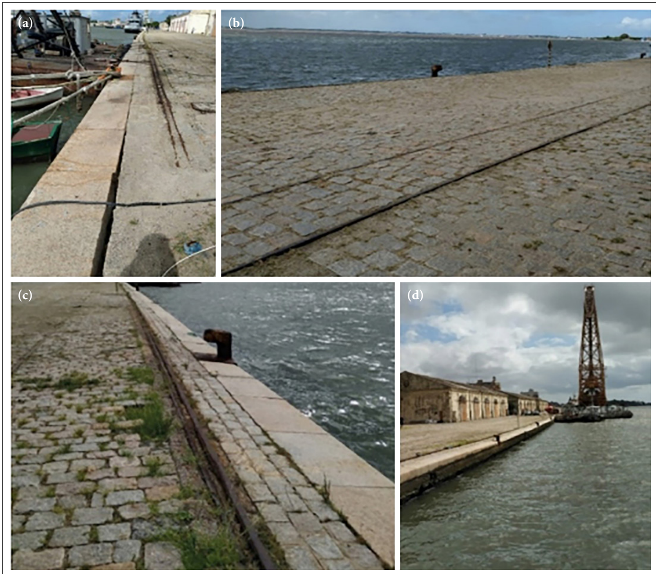
Figure 2. (a) Displacement of the pier structure blocks. (b) Height variation along the pavement and pier crown blocks. (c) Displacement of the gravity wall towards the navigation channel. (d) Area where displacements are most intense.
